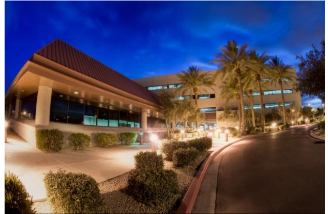
Intel's C7 facility in Chandler is home to several business units focused on product design and development and validation labs.
